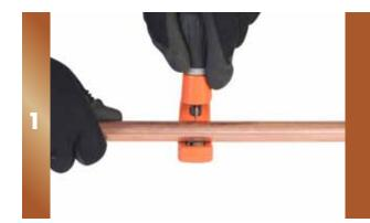
With the use of a tube cutter, cut copper tube to the desired length.
