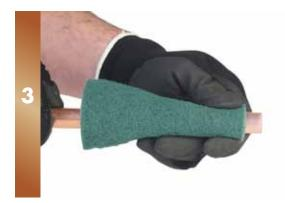
If connecting to existing copper tube to AS1432. Ensure tube is clean by way of soft scourer or emery paper.
