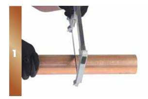
Using a fine tooth saw or tube cutter, cut copper tube to the desired length.
