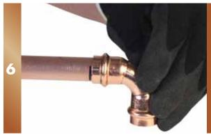
When tube is inserted mark should line up with back of fitting.
