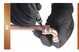
Line up tube with fitting and place a mark on the tube at the correct insertion depth.
