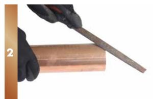
Using a smooth file deburr and clean the end of the tube both internally and externally to minimise turbulence and pressure loss. This will also avoid damage to the O-ring.
