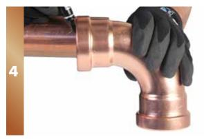
Line up the fitting with the tube and place a mark on the tube at the correct insertion depth.
