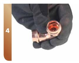
Check that you have the correct fitting for the application. Water will have a black 'O' ring, gas will have a yellow 'O' ring and High temp. will have a red 'O' ring.
