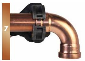
Place the collar over the fitting and check that the fitting sits squarely inside the pressing area of collar.
