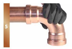
Place fitting onto tube ensuring the mark on the tube lines up with the outer edge of the fitting.
