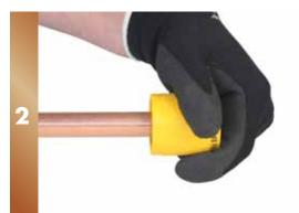
Next using a deburring tool, deburr the end of the tube that will be inserted into the fitting.
