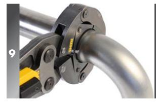
Place the adaptor jaw over the pins on the collar, check that the fitting is still matching up to the insertion depth mark on the tube. Press the trigger on the tool and hold down until piston retracts. Remove the adaptor jaw from the collar, then the collar from the fitting.
